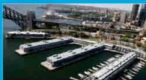
Walsh Bay Apartments
