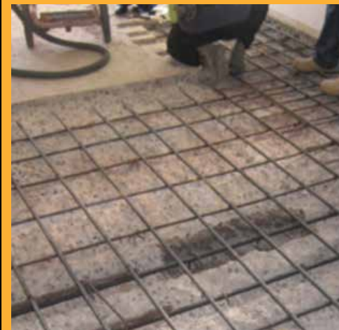
New rebar installation
