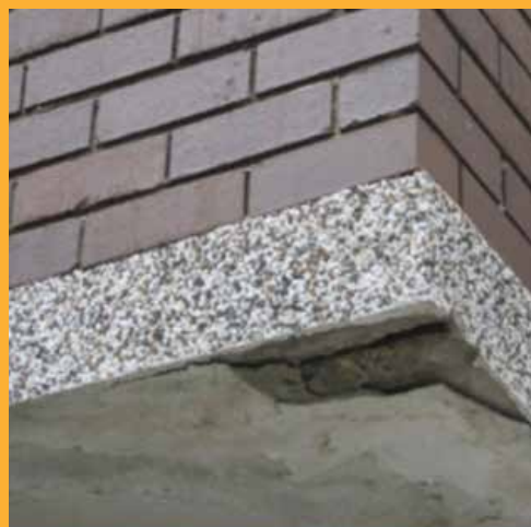
Concrete spalling to soffit
