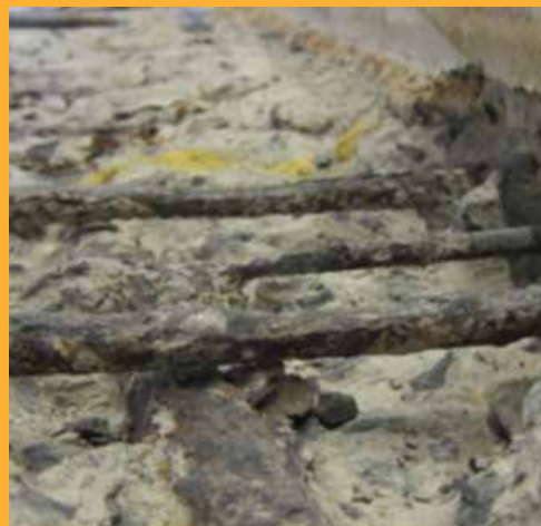
Visible degradation of rebar
