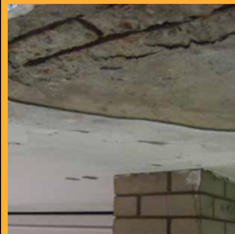
Rusting rebar causes spalling concrete
